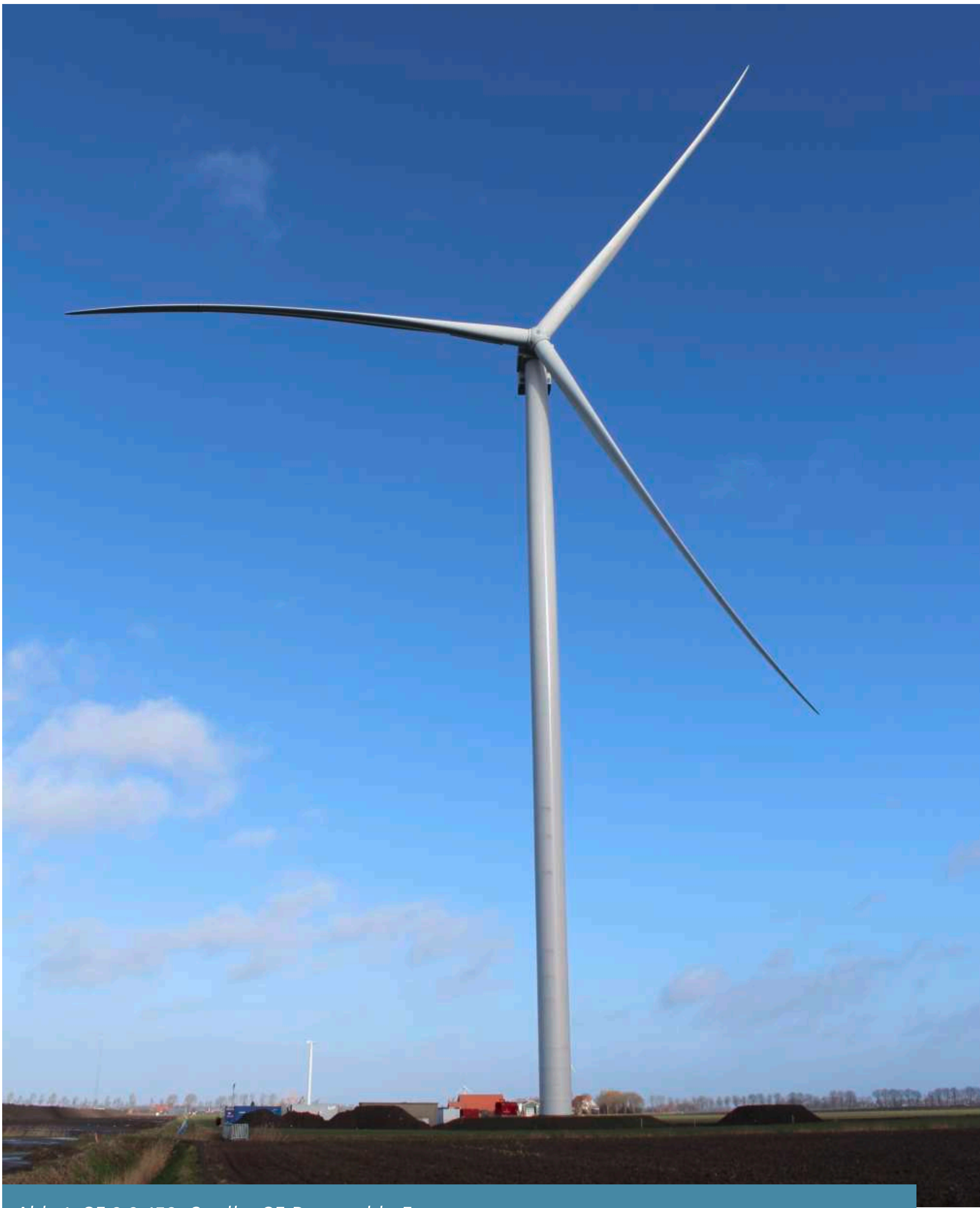
Abb. 1: GE 3.2-158. Quelle: GE Renewable Energy.
